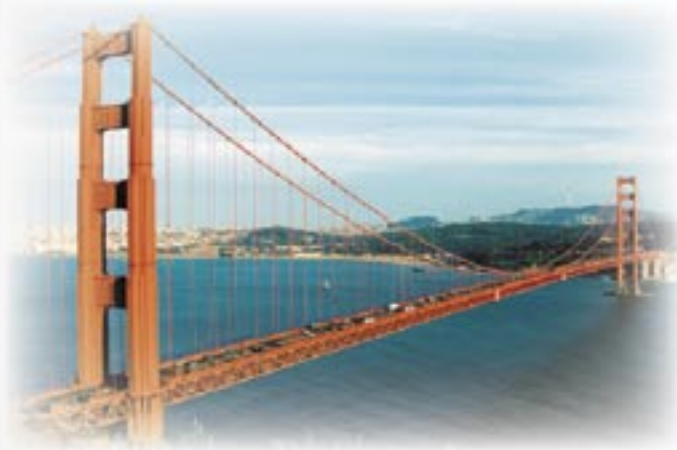
Golden Gate Bridge
